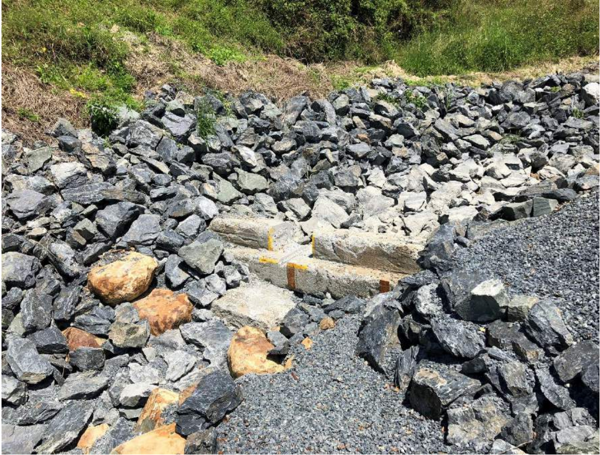
Photograph 17: Check dam constructed along Main Drainage Channel
