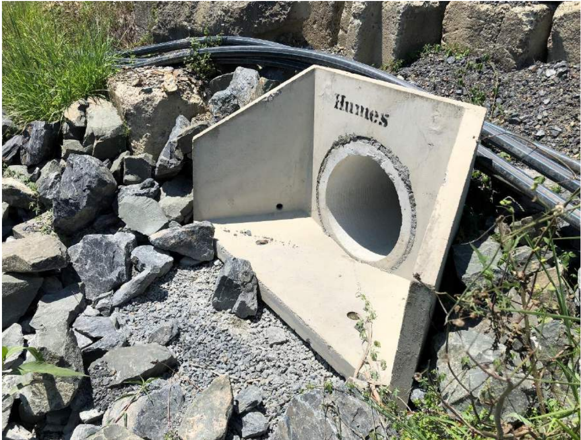
Photograph 3: pipe outlet from Main Dam
