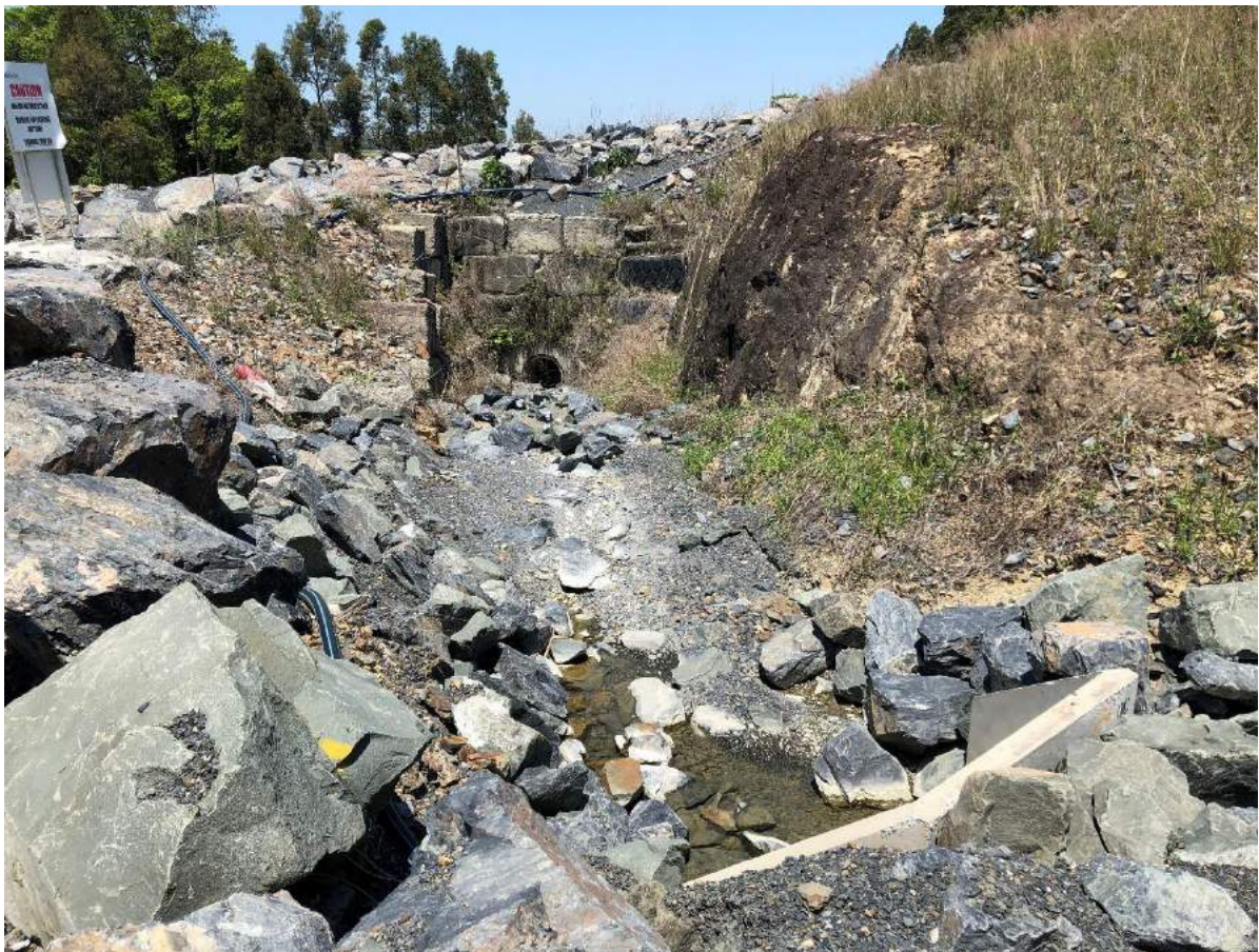
Photograph 4: open channel reach downstream of Main Dam, upstream of access track crossing
