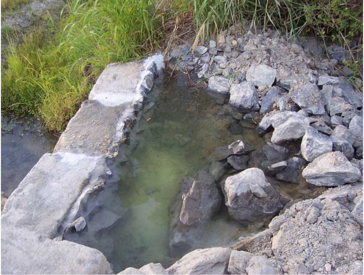
Photograph 19: Concrete lining of Main Drainage Channel immediately upstream of the LDP
