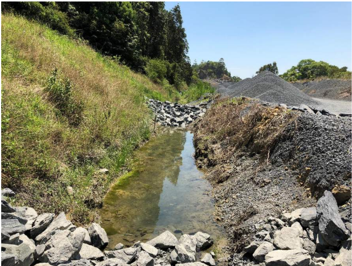
Photograph 16: Check dam constructed along Main Drainage Channel
